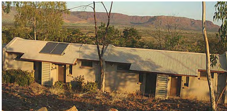
Plate 6: Accommodation quarters at the main Argyle camp
