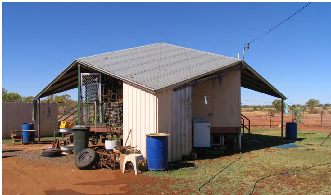
Figure 35: The rainwater collection systems built by a tenant at his Dajarra house provided the main supply of drinking water in 2008. The town bore water was used liberally to maintain a lawn, which reduced dust around the house. (Photo by Tim O'Rourke)
