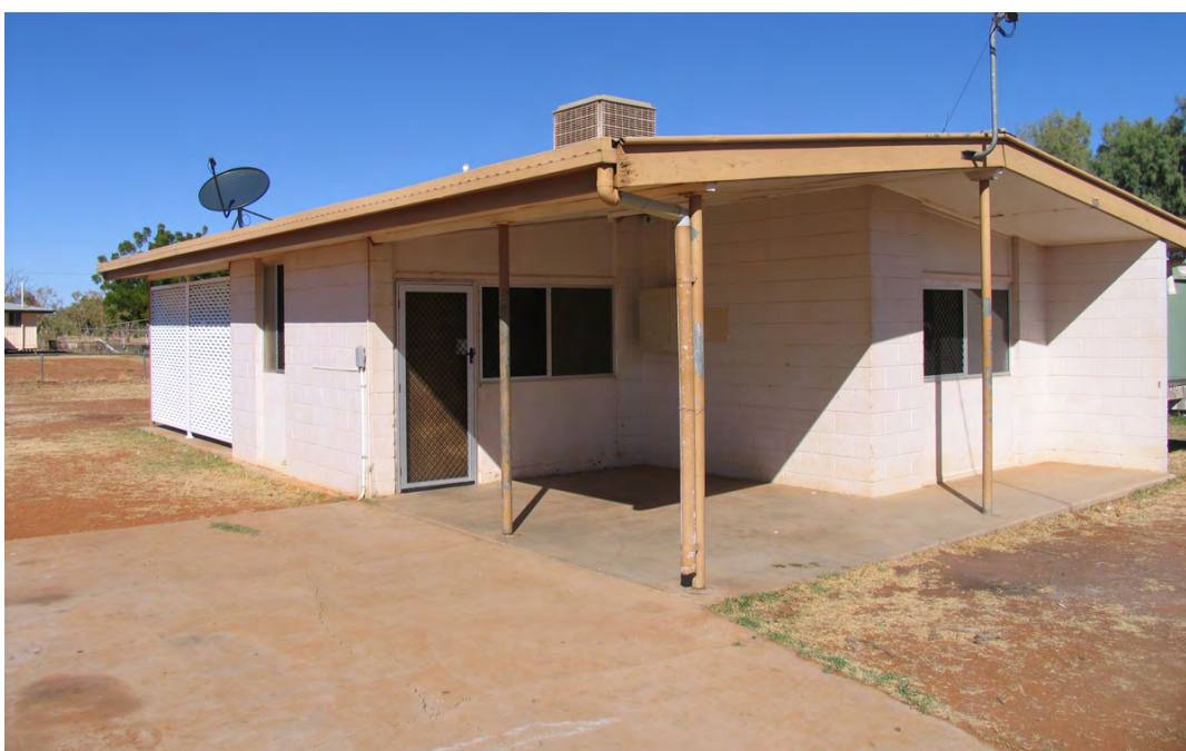
Figure 36: Managed by the Queensland Government, this house in Dajarra was vacant in June 2008. It had been inundated by creek flooding the previous year, with the tenants moving to the Jimberella Hall. (Photo by Tim O'Rourke)
