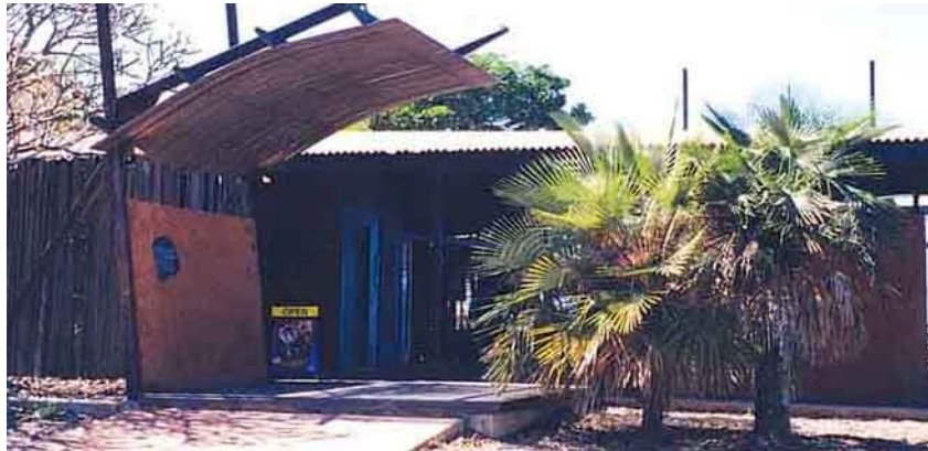
Plate 2: Entrance to the Western Cape Cultural Centre at Evan's Landing near Weipa
