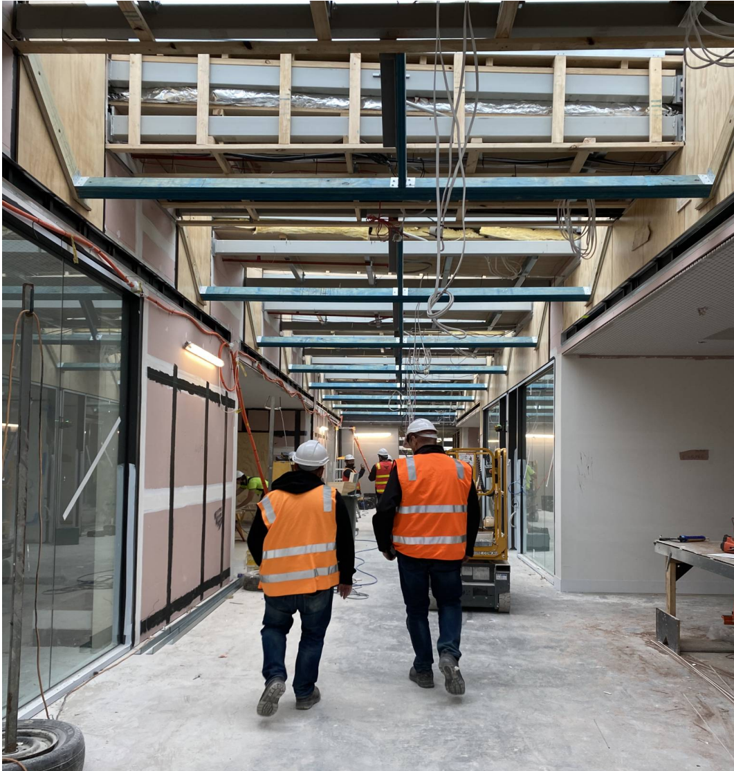
Architectus: Student Hub Site Visit
