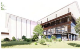
View from Courtyard
